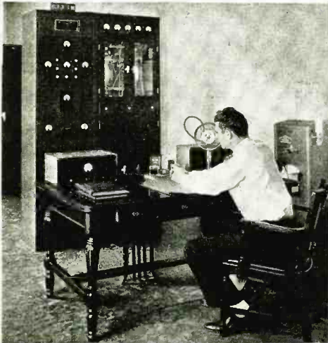
WESTERN ELECTRIC ultra high frequency Police Radio Transmitter, Station W2XEM, Newark, N. J.
