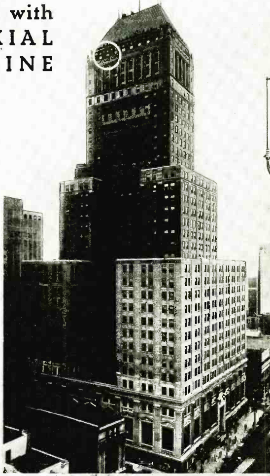
National Newark and Essex Bank Building, Showing location of transmitter and antenna connected by ISOLANTITE COAXIAL TRANSMISSION LINE.
